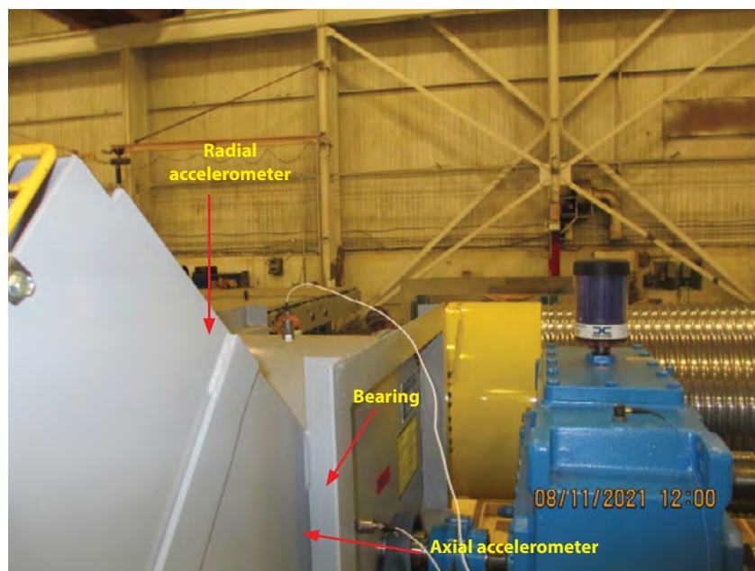
Figure 9: Break Fan Transducer Location during Factory Acceptance Test
